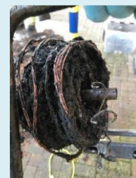
Case of fire ignited by reel-type cable Source: SwindonAdvertiser.co.uk
