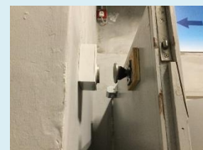
Photo 6: Electromagnetic door not energized
