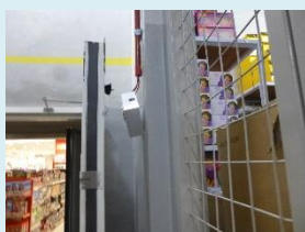
Photo 4: Faulty electromagnetic holder
