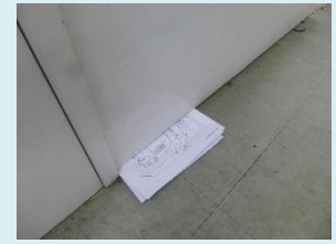
Photo 9 & 10: Checking the gap between fire door and floor
