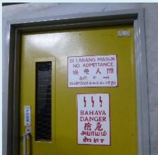
Photo 2: Missing door handle Source: author's past surveys
