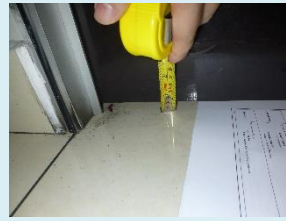
Photo 9 & 10: Checking the gap between fire door and floor
