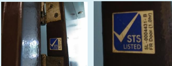
Photo 1: Example of certified fire-rated door Source: author's past surveys
