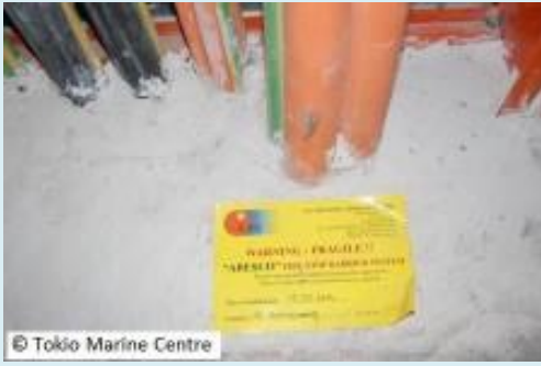
Figure 4: Fire-stopping of penetrations
